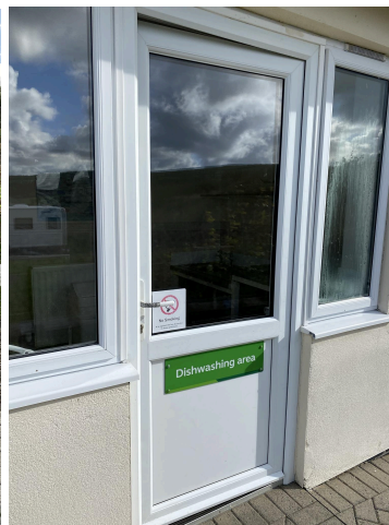
Entrance to dishwashing area
