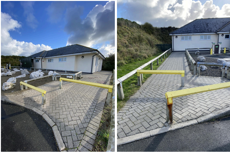
Ramped entrances to the toilet block
