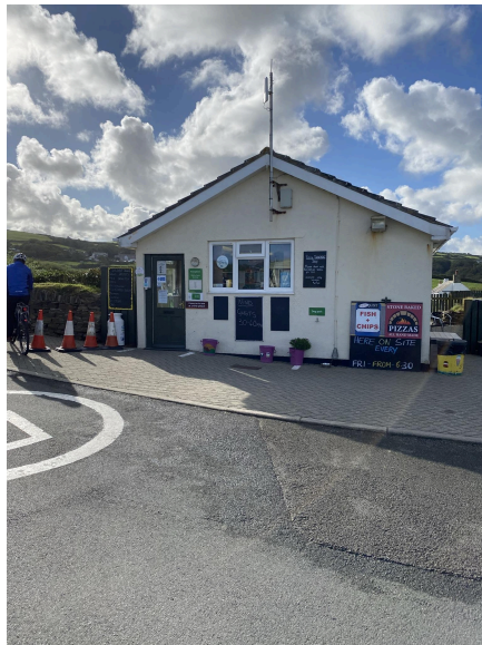
Reception Entrance via a dropped kerb
