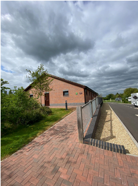
Ramp to Toilet Block
