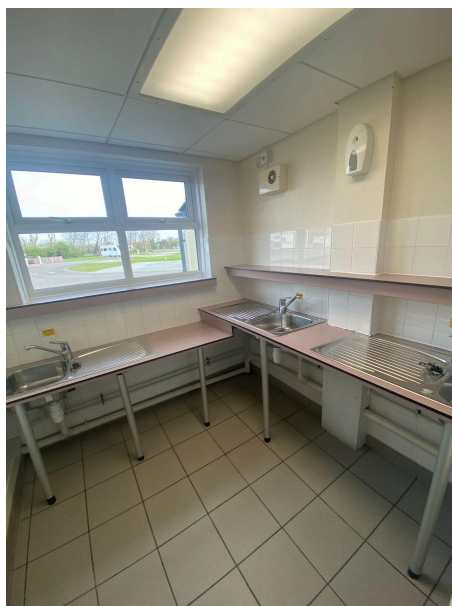
Dishwashing Area - Toilet Block 1
