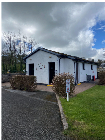
Annex Toilet Block
