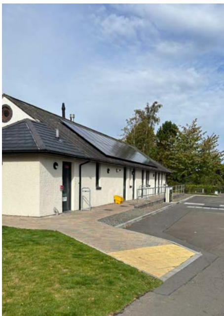
Toilet Block B
