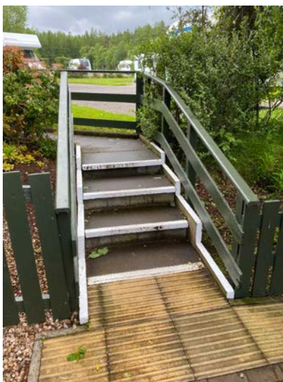
Steps to the back of the building
