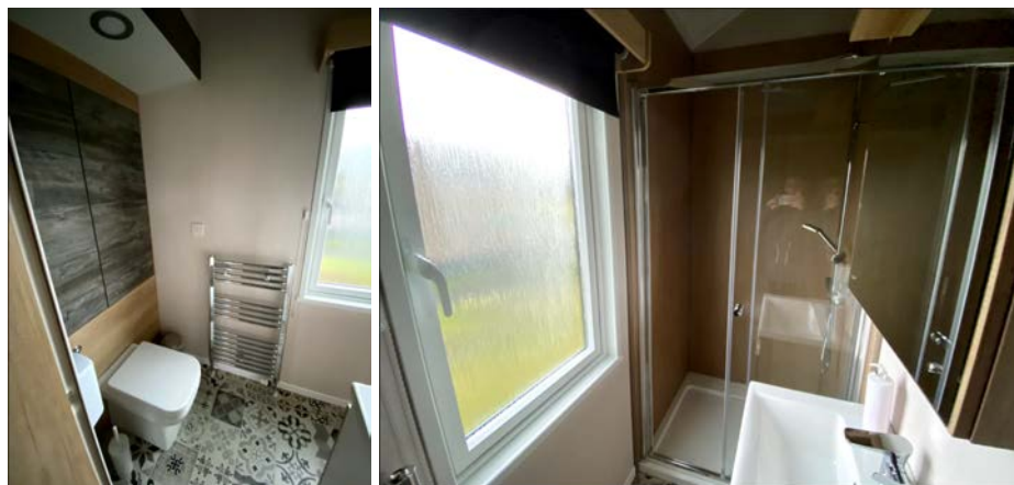
The bathroom is at the back of the cabin, and narrows to 560mm wide between the sink and the wall.
