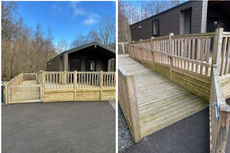
Ramped access to the glamping pod
