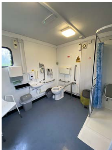
Accessible Toilet and Shower
