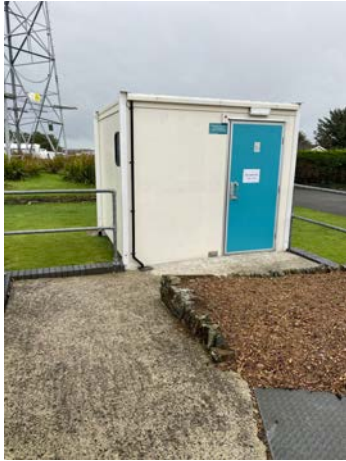
The Accessible Cubicle
