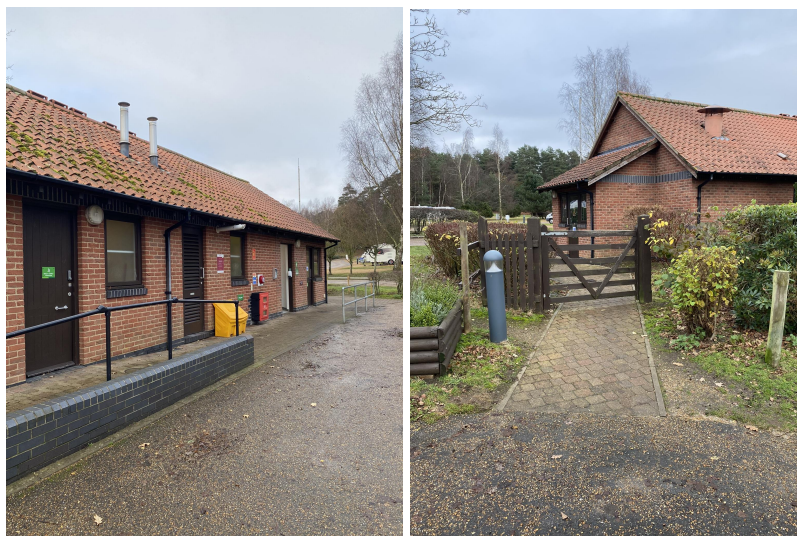
Access to Toilet Block 1
