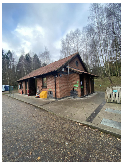
Access to Toilet Block 2
