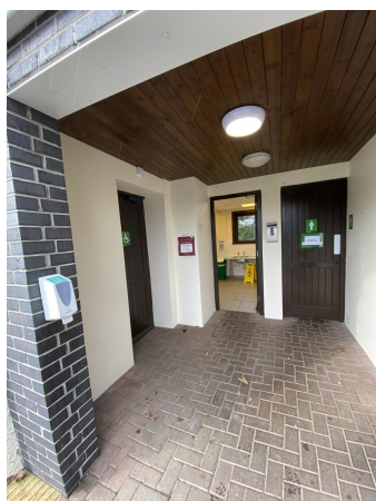
Alcove to Accessible WC and Shower Cubicle
